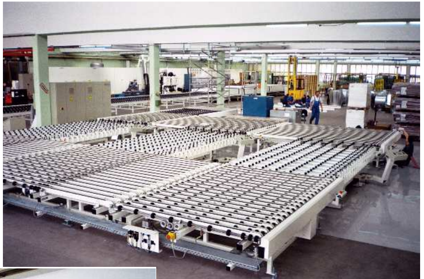
Flachglas-Förderanlage Flat glass-conveying plant
